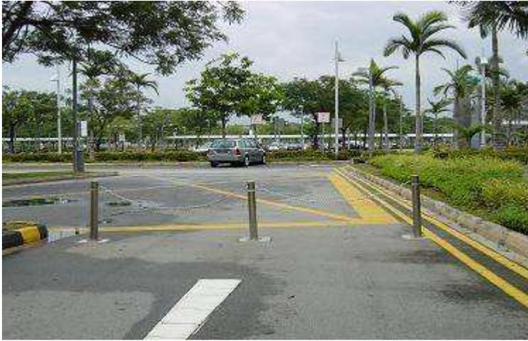
The picture on the left illustrates an example of how accessible features are rendered un-useable. The driveway is meant as a passageway for wheelchair users. However, to avoid other car drivers from using the passageway as well, chains have been erected across the bollards. This impedes wheelchair users from using the passageway.
