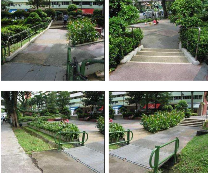
A typical example of an inter-connectivity issue is the difference in levels. There is no continuous ramp constructed to link between the precinct space and the pedestrian walkway along the main road. It is difficult for a wheelchair user to reach the main road.
